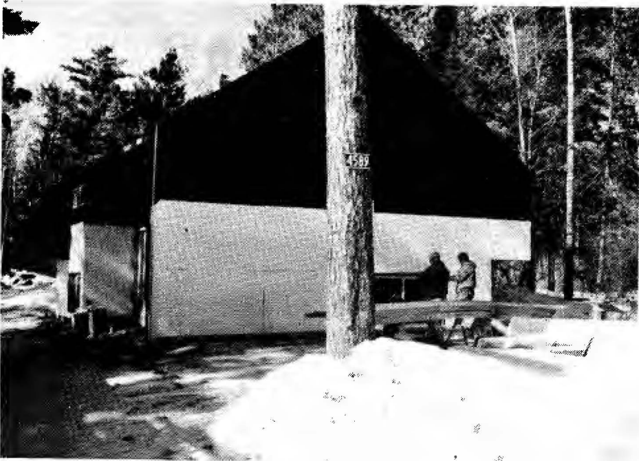
'Bird' house being remodeled in Palmquist
