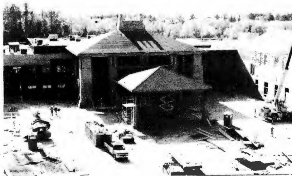
Front view while still under construction.
