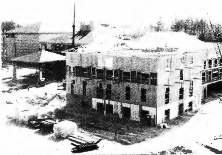
Hotel . . . while still under construction.
