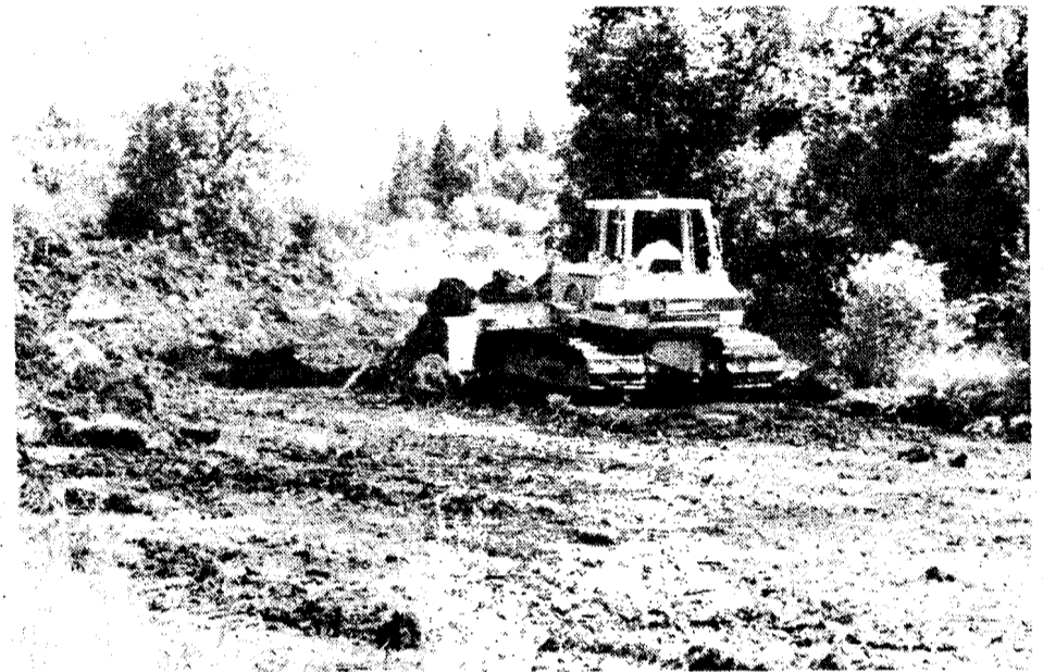
Work starts on the new commod building.
