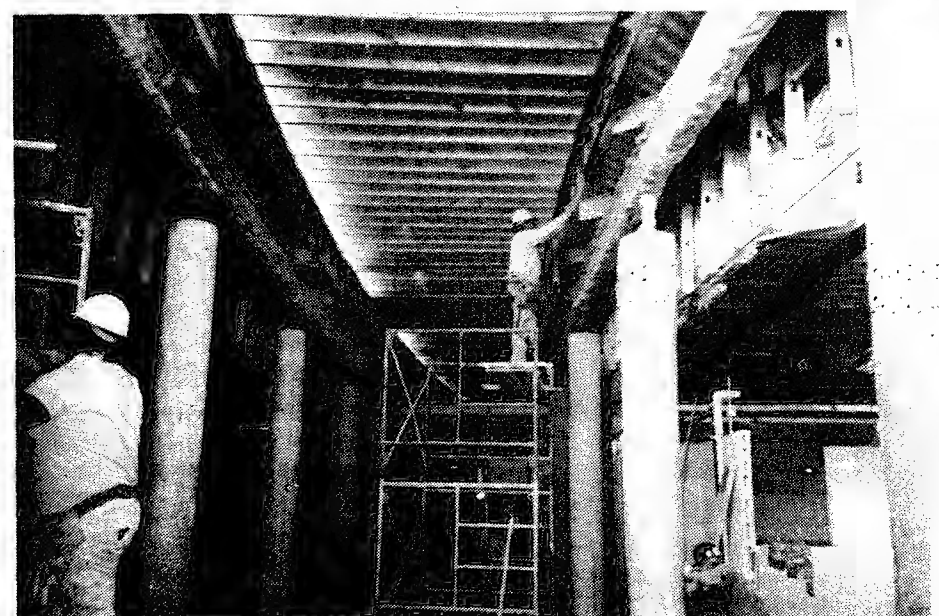
This view shows workers in the main hallway. Note the space above. This will be the future skylight.
