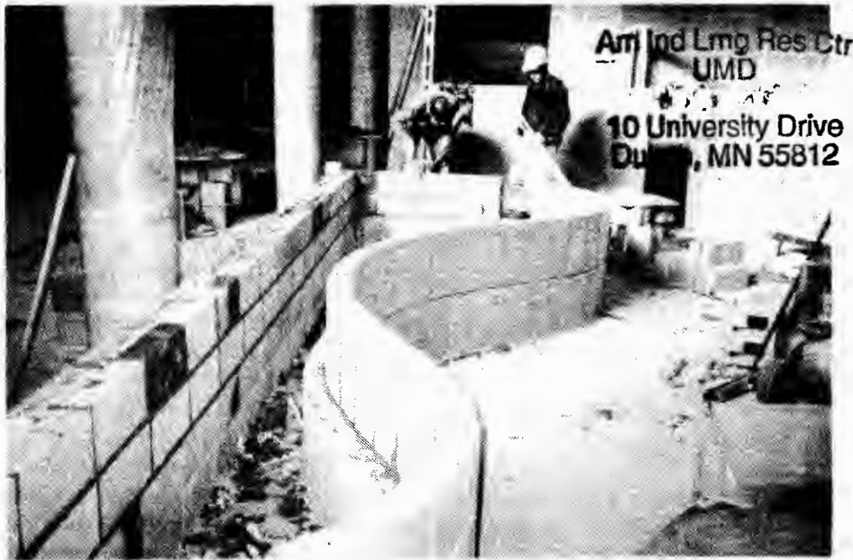
Masonry workers laying block on interior planter.
