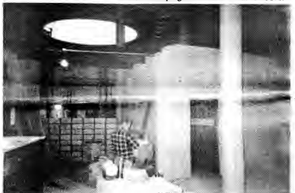
This shows the skylight in the main building.
